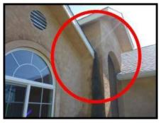
In this case, the issue is lack of proper kick out flashing and roof to wall flashing.
